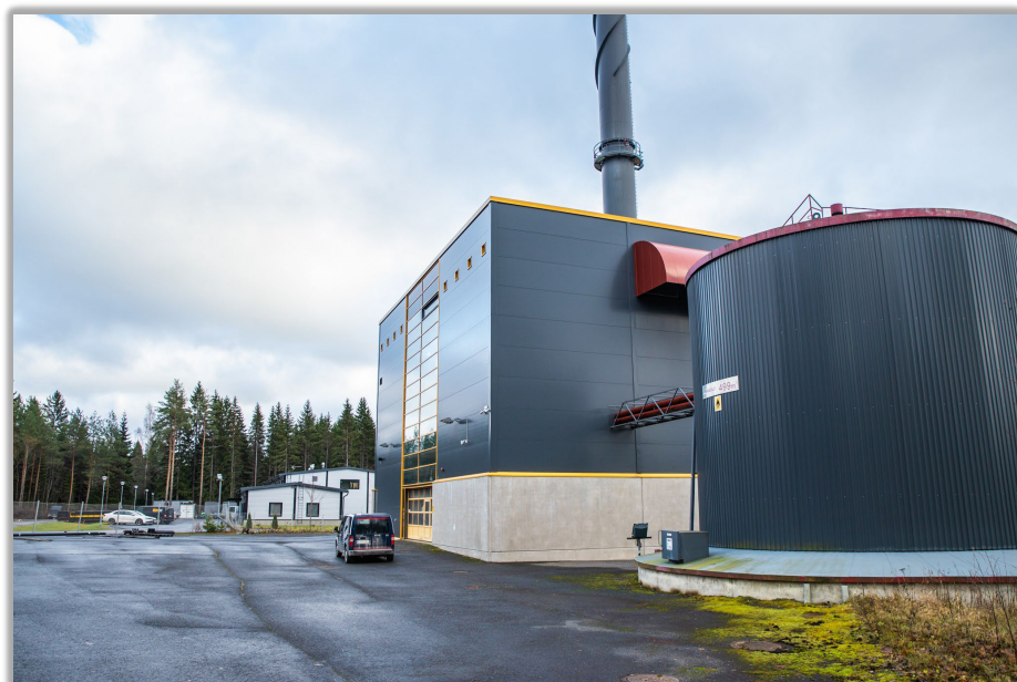
Rokkala reserve heating plant has a capacity of 40 MW.
