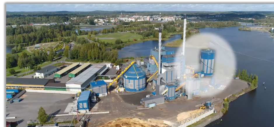
Heat accumulator carries 7,000 m 3 of water and is utilized in production optimization. The capacity of the accumulator is 350 MWh.
